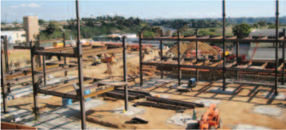
Using the Design-Assist project delivery method, McCarthy Building Companies is constructing the 279,000 sq. ft. Acute Care Pavilion at Rady Children's Hospital and Health Center near San Diego. The project is slated for completion in the spring of 2010. McCarthy also had previously completed design-build services for an adjacent 1,000-car parking structure including a podium deck for the future new Ronald McDonald House.
